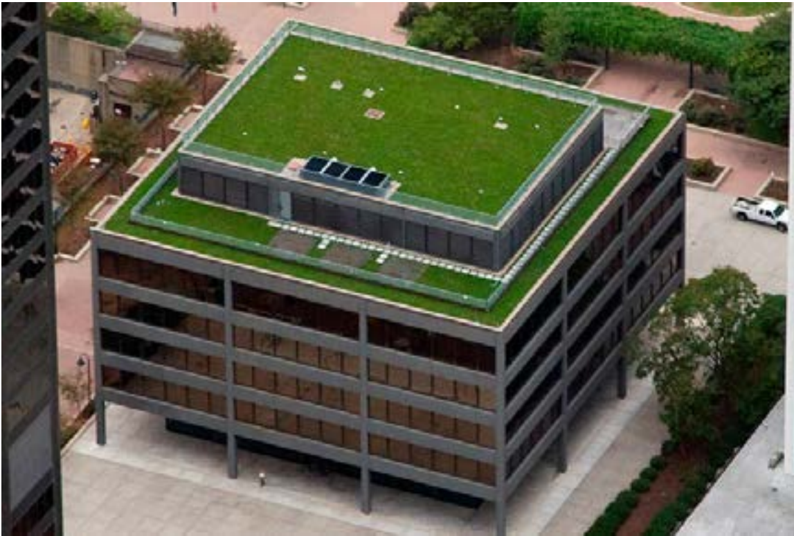
Green roof installed atop the American Life building in Downtown Louisville.
